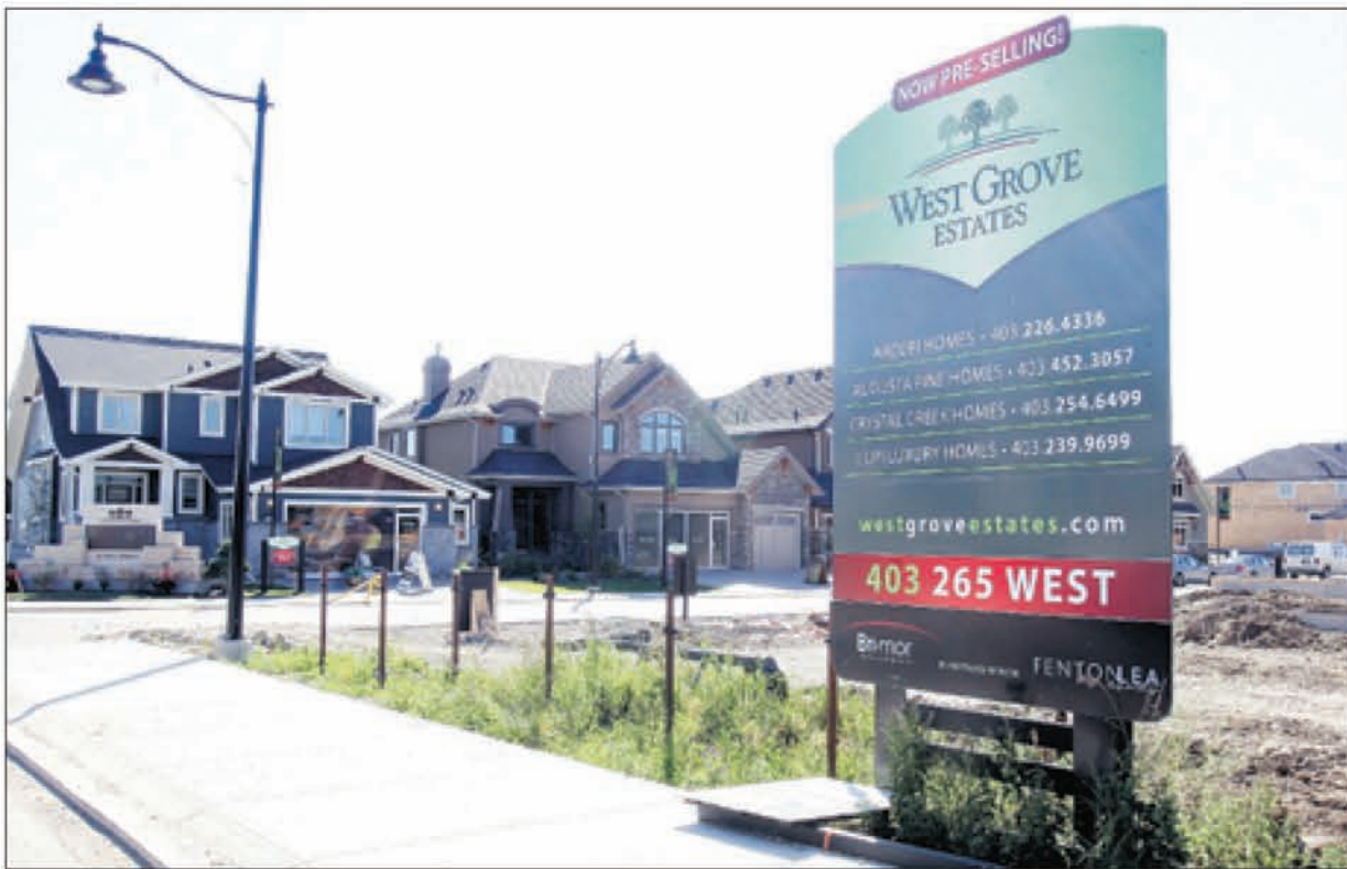
Construction work is being undertaken in the Bri-Mor Developments project next to the parade of showhomes for the West Grove Estates community. Dean Bicknell, Calgary Herald
